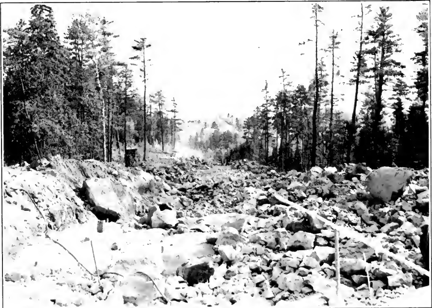
Grading, Highway No. 11 – Rock Cut near Herridge Lake, Timagami Park
